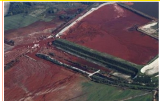
Photo shows the damaged reservoir near an alumina plant, seen from the air in Kolontar, 150 km (93.2 miles) west of Budapest
