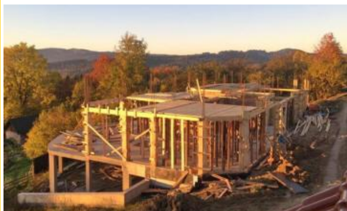
Centre of Light phase 2 construction, completing the wooden structure and roof.
